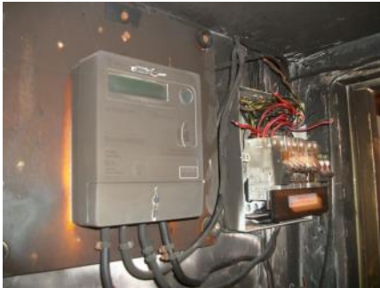
Fire damaged electrics will require replacement
